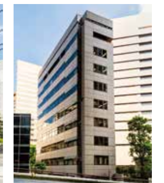
Kintetsu Kasumigaseki Building (Chiyoda City, Tokyo) 4 minutes' walk from Kokkai-gijidomae Station on the Tokyo Metro Chiyoda Line and Marunouchi Line; 5 minutes' walk from Tameike-Sanno Station on the Tokyo Metro Ginza Line and Namboku Line
