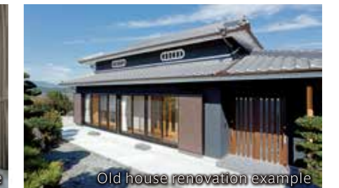
Old house renovation example
