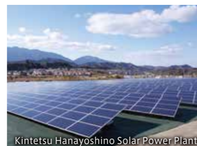
Kintetsu Hanayoshino Solar Power Plant
